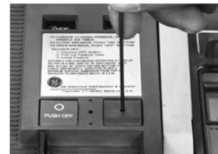
Activating the breaker closing mechanism through the hole in the Hidden "ON" Button
